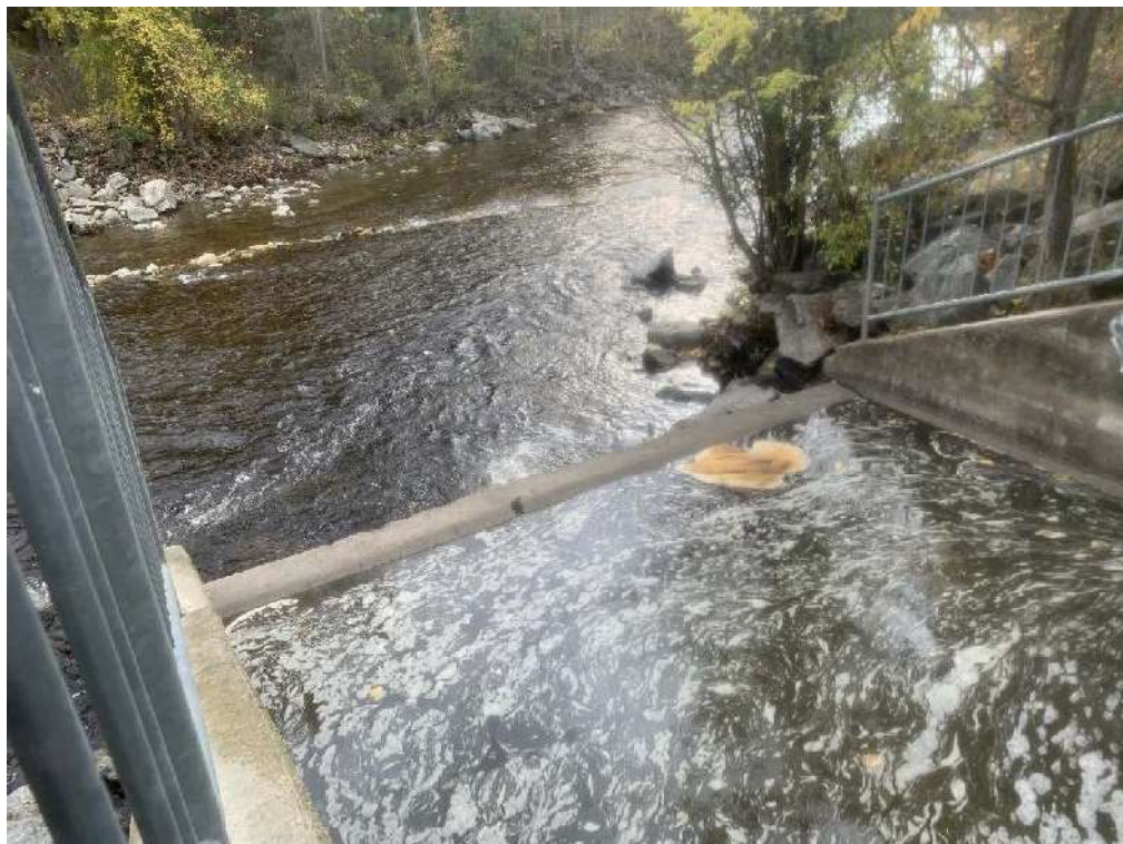
Appendix Photo 8. Downstream view of diversion outfall into Mission Creek.
