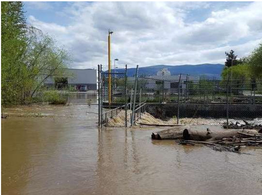
Appendix Photo 6. View south (right bank to left bank) of Mill Creek diversion structure during May 2017 flood obtained from online search. Grizzly structure and walkway visible in photo centre and diversion inlet to right of center within fencing.
