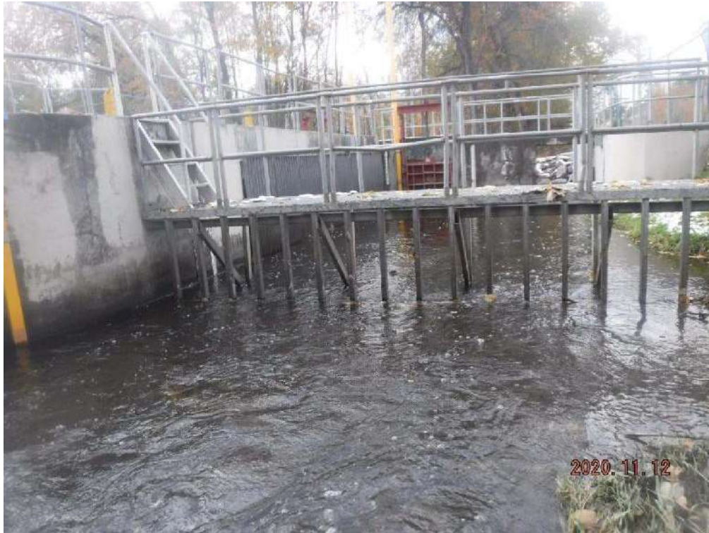
Appendix Photo 1. View (downstream) of the diversion structure.
