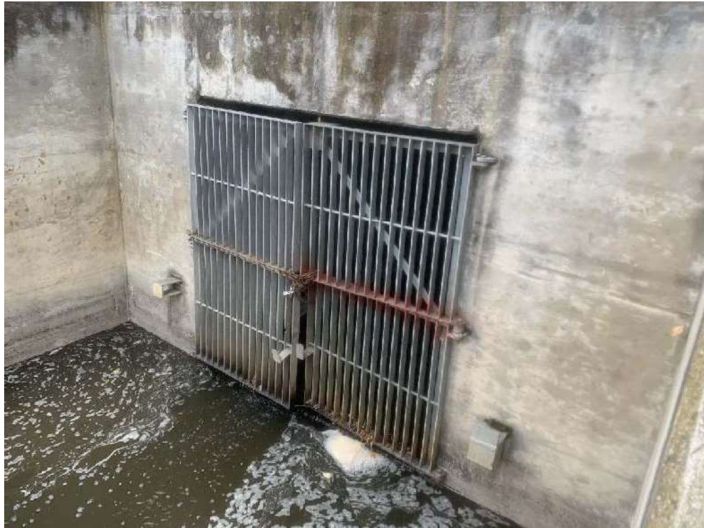
Appendix Photo 7. View of diversion culvert outlet at Mission Creek.
